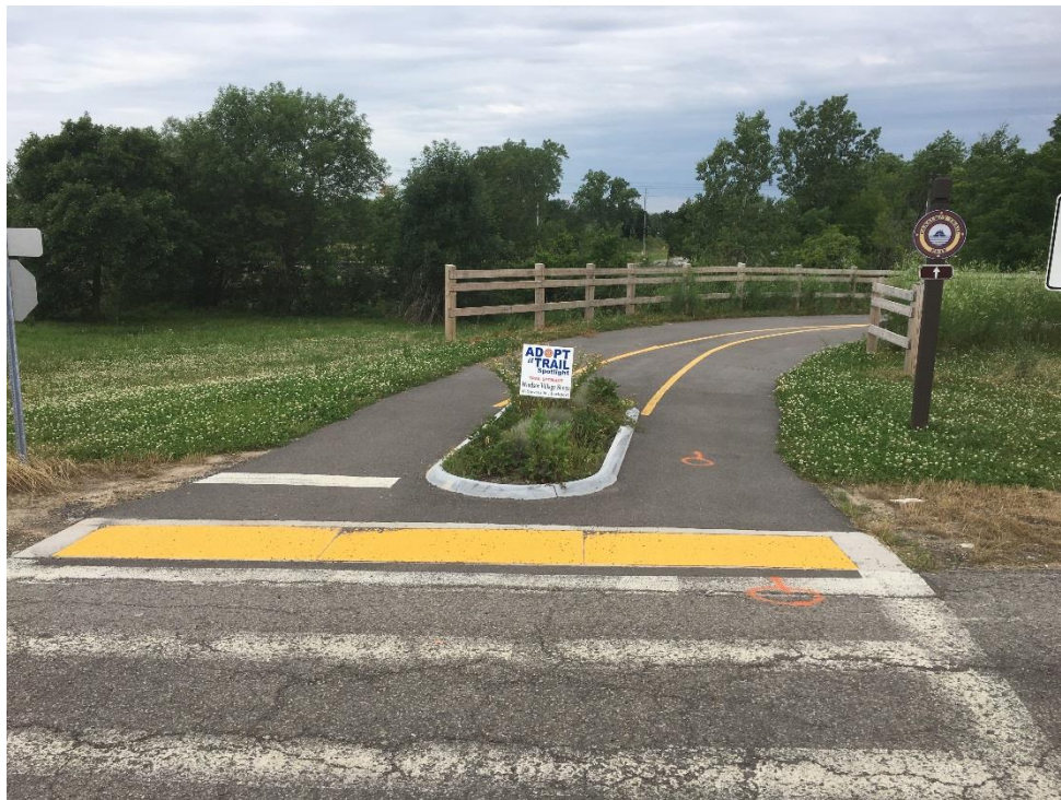
Above: Typical road crossing on the newly constructed Albany-Helderberg Rail-Trail in Albany County. Below: Emergency vehicles can drive over the low island at this Erie Canalway Trail road crossing.
